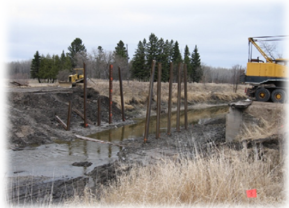
Figure 2. CR7 Bridge demolition and construction
