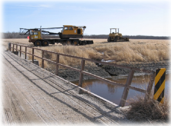
Figure 1. Construction equipment in place to start the replacement of the CR7 Bridge over the Thief River
