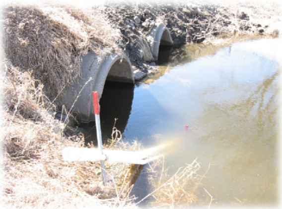
Figure 7. Eureka Midge and HOBO Water Level Logger deployment pipes installed in Heartsville Coulee
